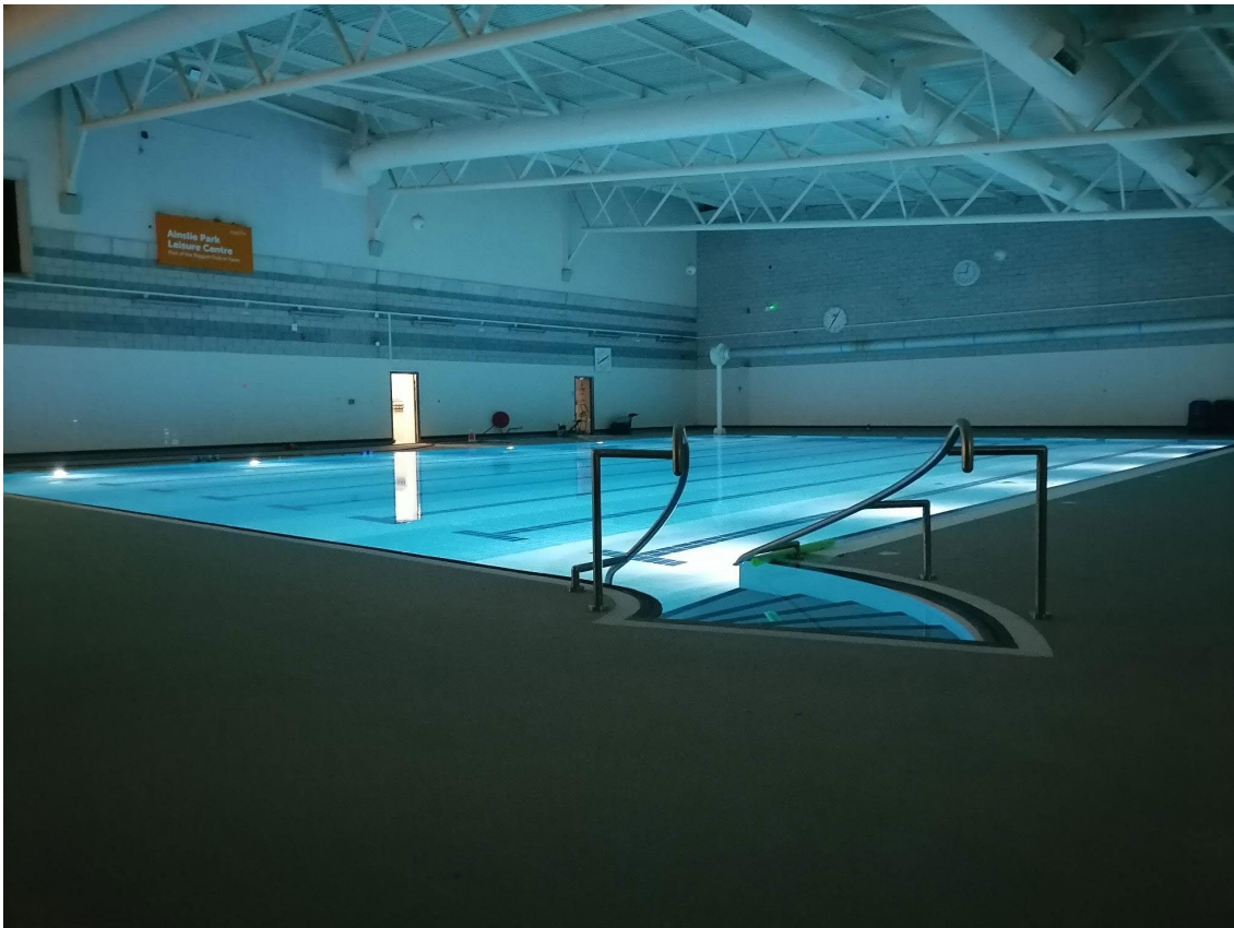
Photograph of Ainslie Park Leisure Centre after swimming pool underwater lighting improvements
