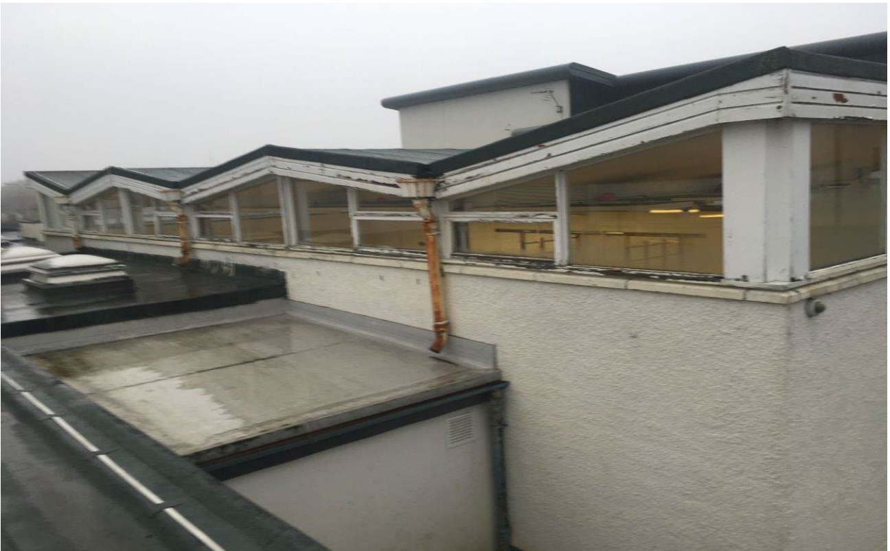
Photograph of windows & cladding at Currie Primary School (Games Hall) before improvements
