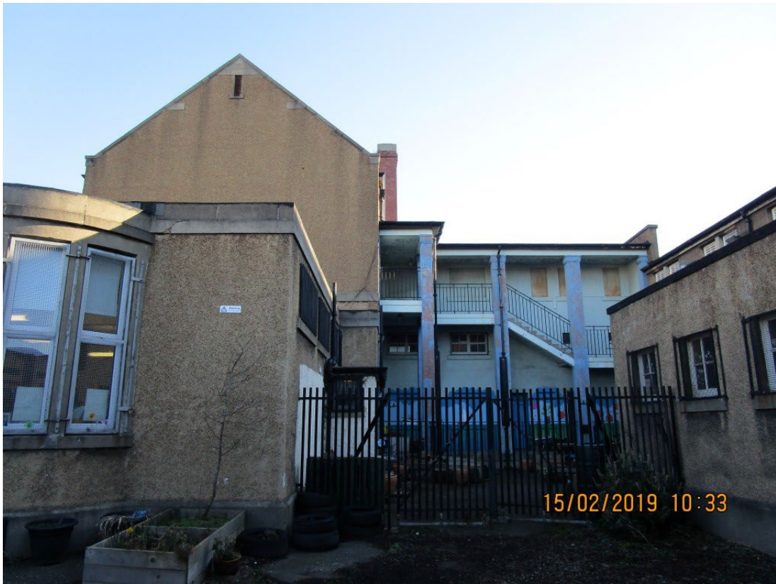
Photograph of Granton Primary School external building fabric & windows before improvements
